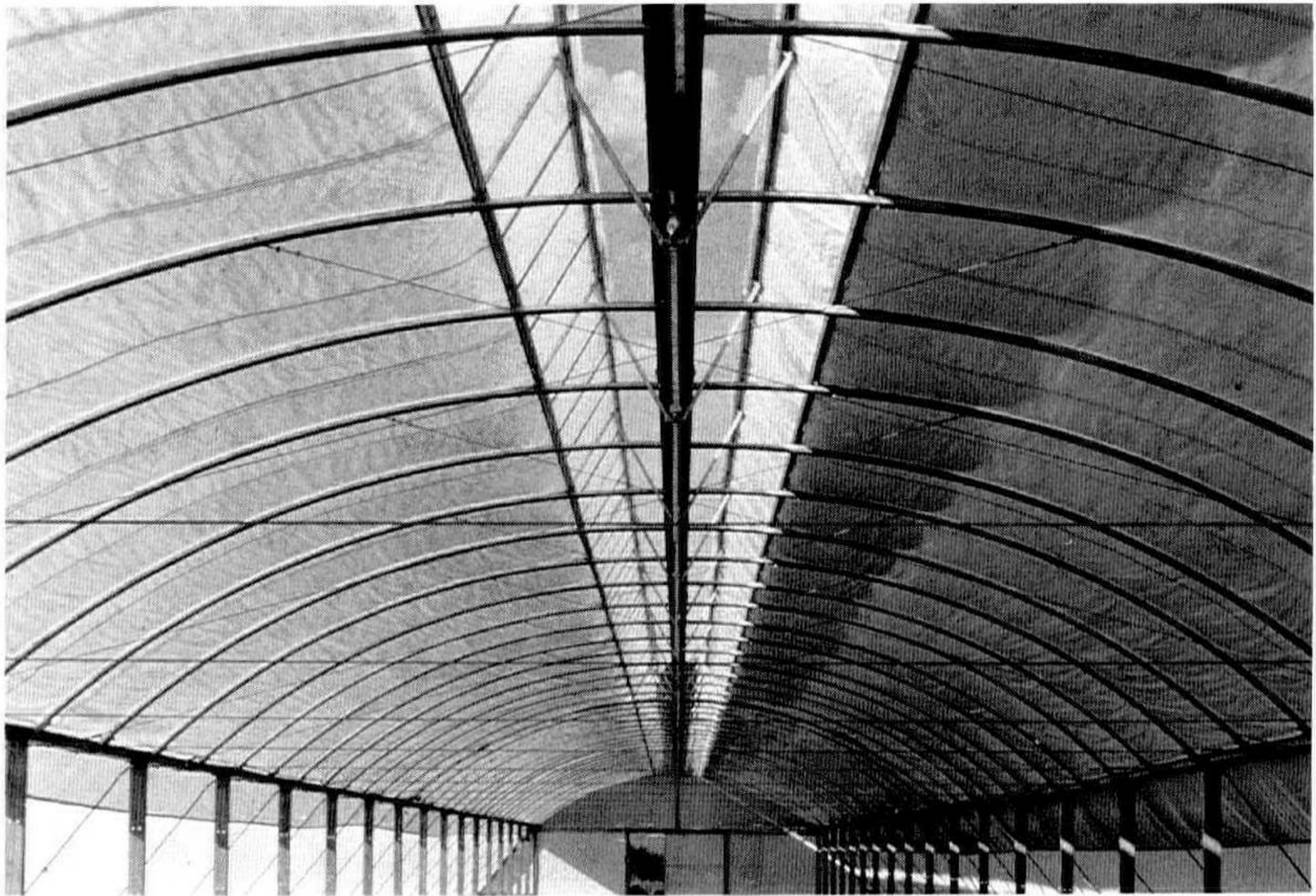
Figure 2. Roof-vented poly-covered quonset structure.
