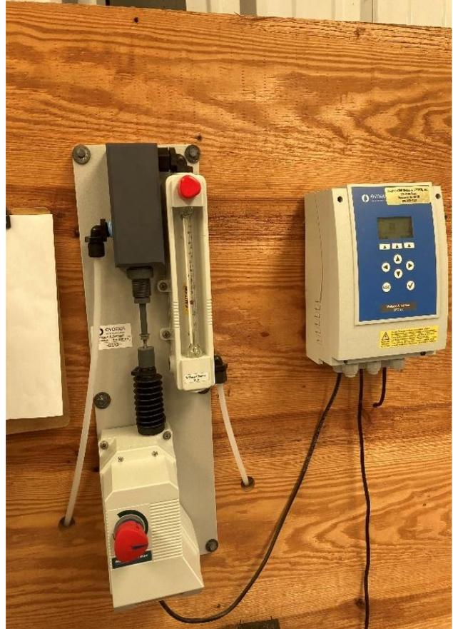
**Figure 17.** (top left) Interior view of pump house, (top right) a Yardney sand filtration system with automatic backflush, (bottom left) chlorine gas cylinders with a regulator, and (bottom right) a Wallace and Tiernan<sup>®</sup> S10k gas feed chlorine metering system.
