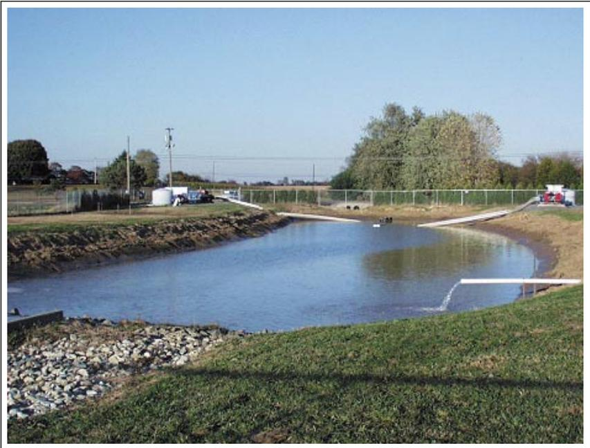
Figure 4. Finished tailwater recovery system.
