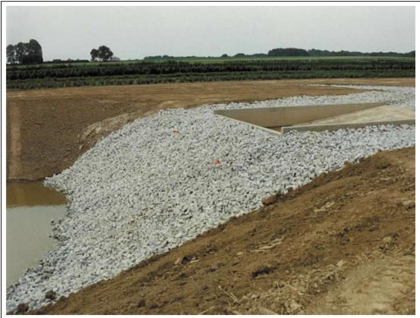
**Figure 2.** Rock layer on the surface of the pond wall below the weir.
