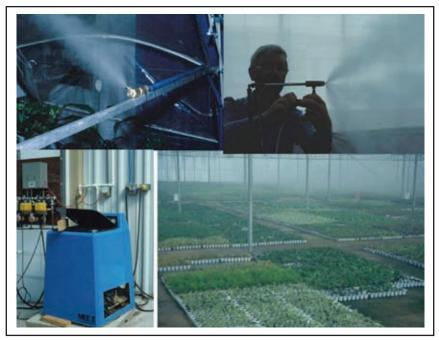
**Figure 4.** Fog systems form fine water droplets with an average size of 15  $\mu$ m. Fog has a high surface: volume ratio, which helps water remain suspended in air as a vapor (gas) to maximize evaporation. Fog does not condense, avoids over-saturation of media and foliar leaching, which occurs with mist.
