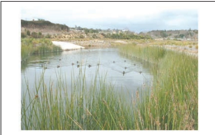
Figure 1. Matua storm water pond 1 year after planting.
