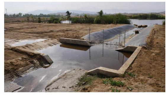
Figure 3. Sediment forebay designed for easy clean out.
