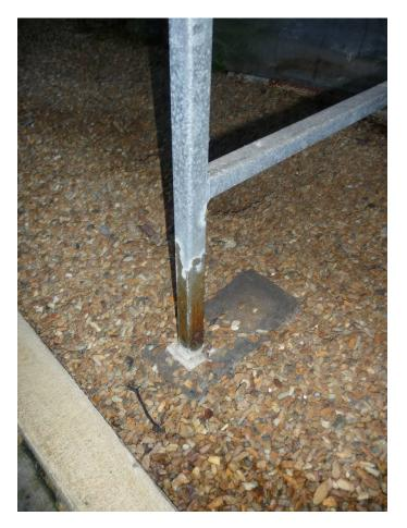
Fig. 10. Water proof grease to stop pests climbing.
