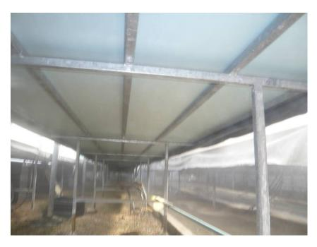
Fig. 7. Module galvanized frame using high density foam for insulation and support.
