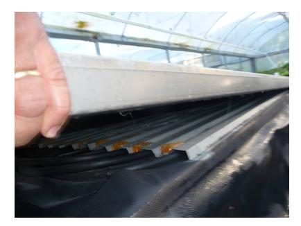
Fig. 9. Single run low pressure poly pipe in steel channels. Spray foam to locate pipe with the bench siting atop.
