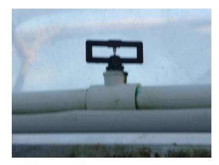
Fig. 5. Enlarged mist nozzles and conventional plumbing at 130 psi.
