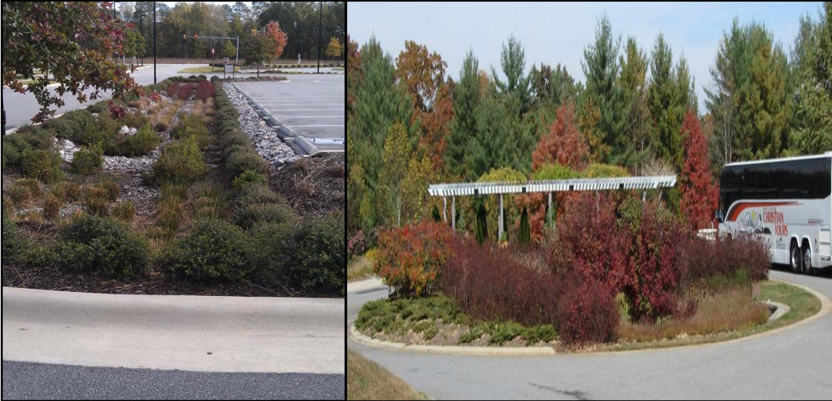
Fig. 1. Two rain gardens in North Carolina [Clayton, NC (left) and Asheville, NC (right)] with different designs, plantings and runoff collection from varying impervious surfaces.
