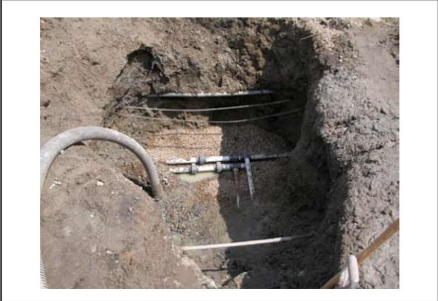
**Figure 6.** Underground clear water and fertilizer mains, which were cut to show algae and biofilm growth in the absence of sunlight.
