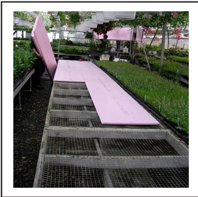
**Figure 10.** Installing bottom insulation in combination with Aquathermat.
