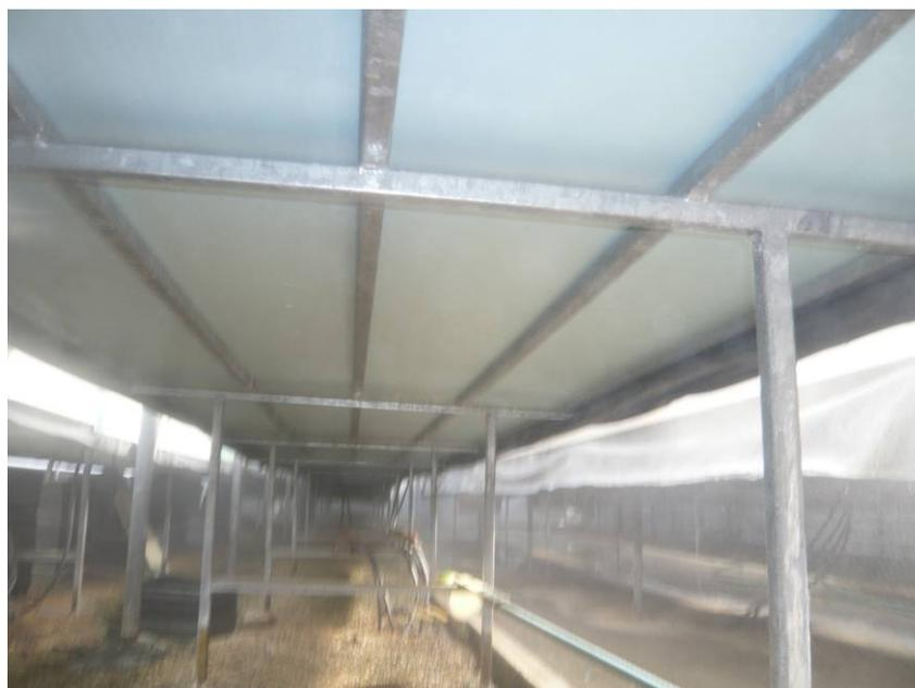
Fig. 7. Module galvanized frame using high density foam for insulation and support.
