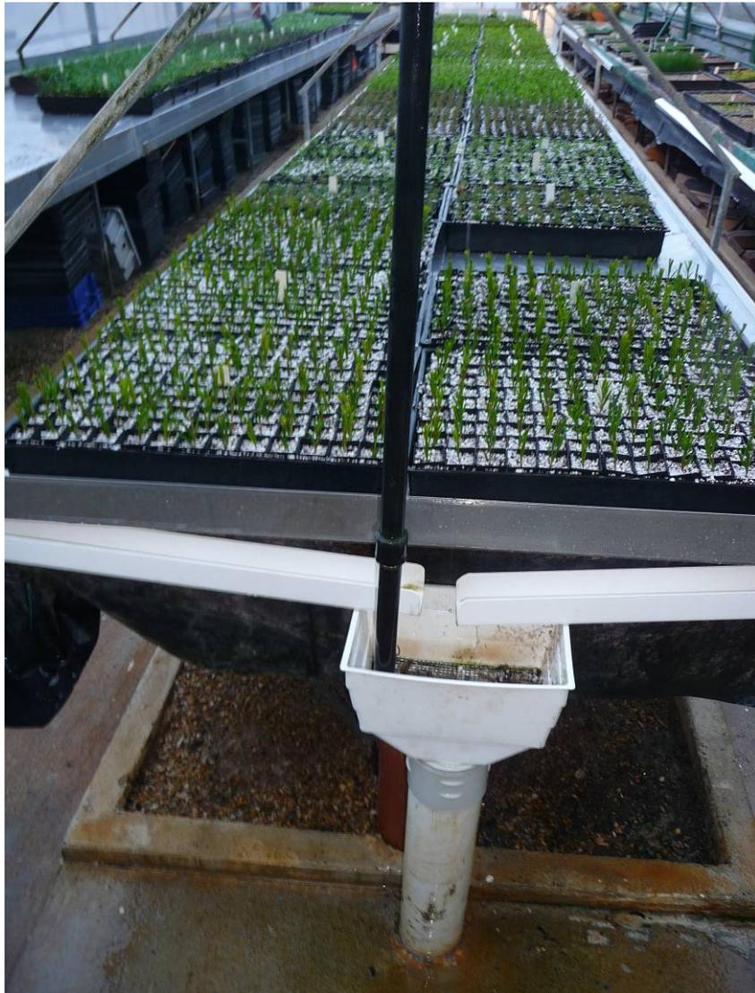
Fig. 11. Our newer system to drain the benches.
