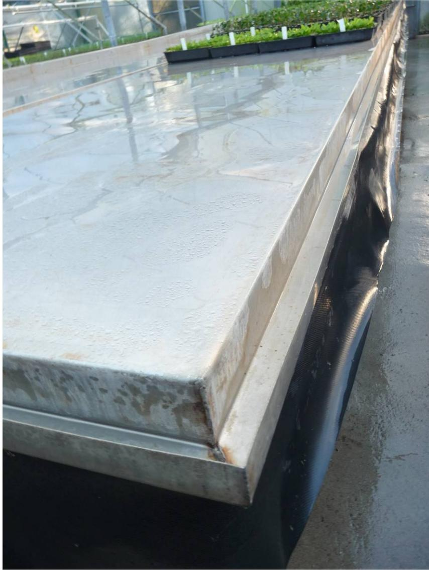
Fig. 8. Stainless-steel benches with side gutters, and plastic side curtains.
