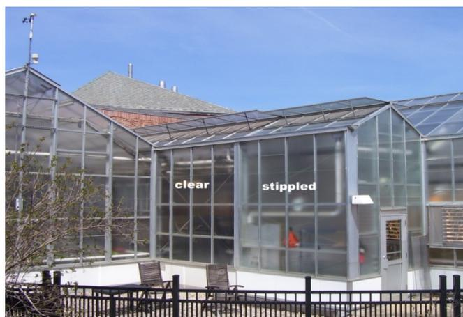
Figure 1. Clear and stippled greenhouse glass.
